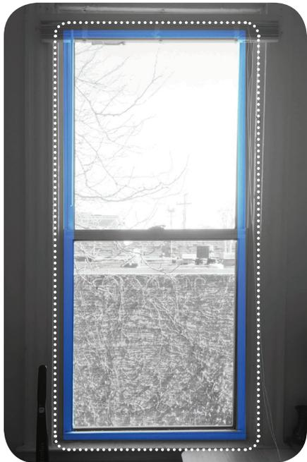
**Weatherstripping will be applied to all sides of the windows, the top of the upper window, and the bottom of the lower window.**
